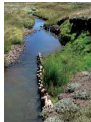
Comanche Creek bank stabilization using post vane structures to move the main flow away from an eroding bank while building a new bankfull bench. Left, July 2006, right, September 2010. Photo view looking upstream.
