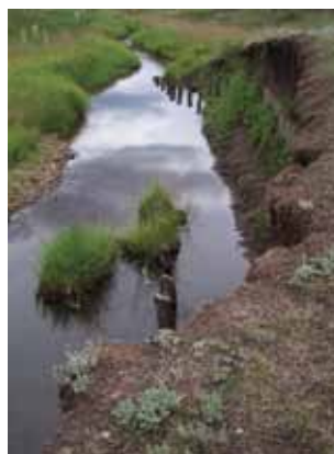
Comanche Creek bank stabilization using post vane structures to move the main flow away from an eroding bank while building a new bankfull bench. Left, July 2006, right, September 2010. Photo view looking upstream.
