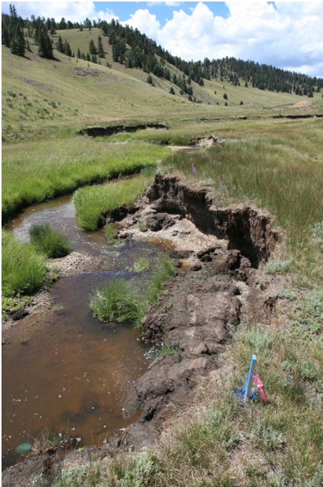
A legacy of heavy use in the Comanche Creek watershed has caused stream banks to become unstable, causing increased sedimentation. Photo by Courtney White
